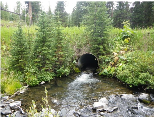
Figure 22: Wolverine Creek culvert on USFS Road 237.
