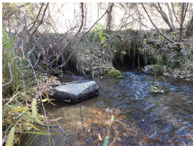
Figure 41: Two culvert system on Rumbaugh Creek.
