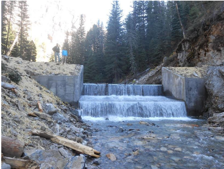
Figure 38: Cabin Creek Barrier.
