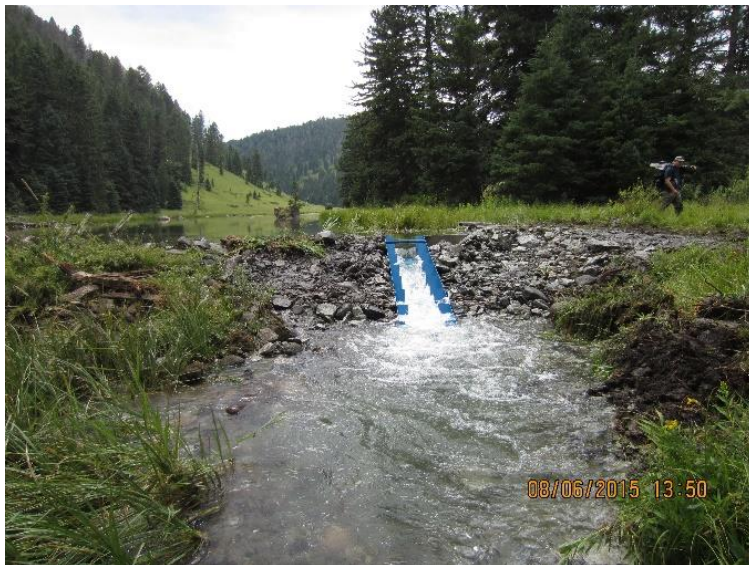
Figure 27: Smith Lake fish ladder.
