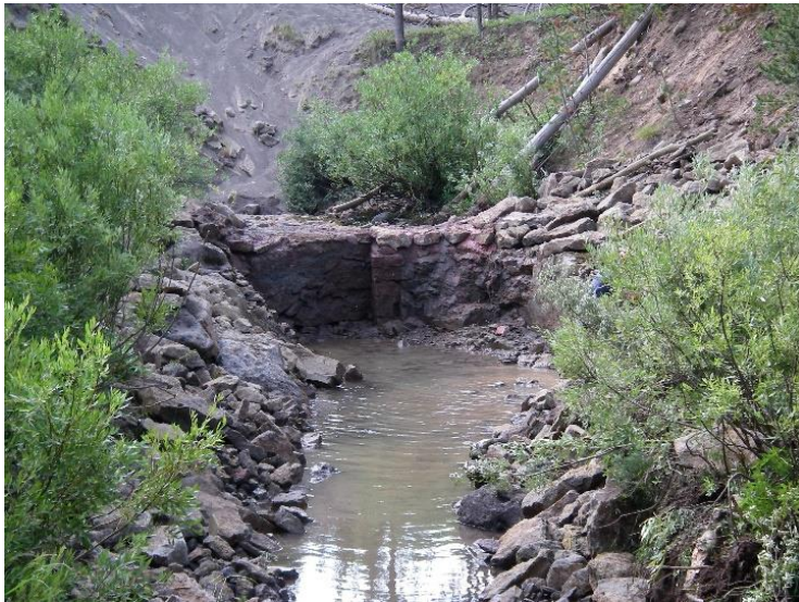
Figure 49: Improved barrier structure on the Upper South Fork Madison
