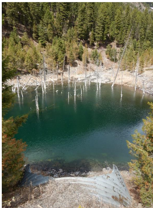
Figure 34: Rock Creek pond at MT Highway 287 culvert crossing.
