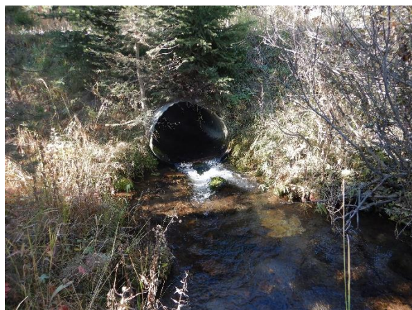
Figure 42: Downstream culvert on Cherry Creek.
