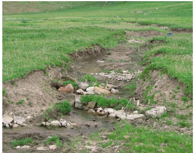
Figure 10: Horse Creek baffle installation in 2006.
