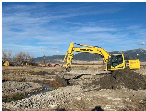
Figure 14: Construction of New Moore Creek Stream Channel
