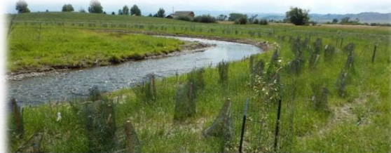
Figure 11: Large bend on part of Lower Jack Creek Restoration. Note the spillover of high water onto banks that soaked into the riparian area and provided water for soil recharge and establishing plants during the project's first year.
