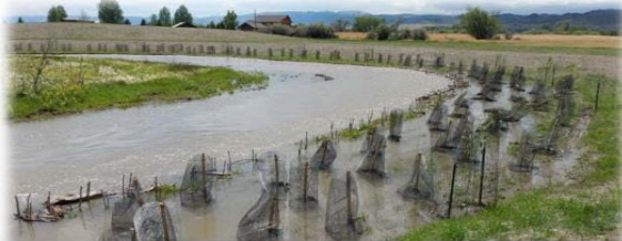
Figure 11: Large bend on part of Lower Jack Creek Restoration. Note the spillover of high water onto banks that soaked into the riparian area and provided water for soil recharge and establishing plants during the project's first year.
